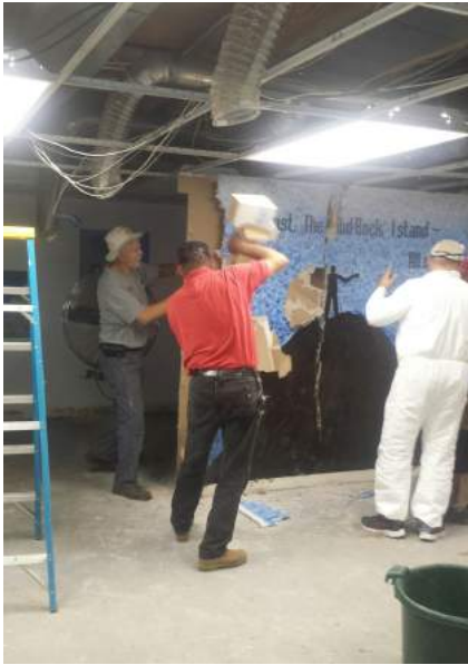
Non-load-bearing partitions were demolished and removed.
