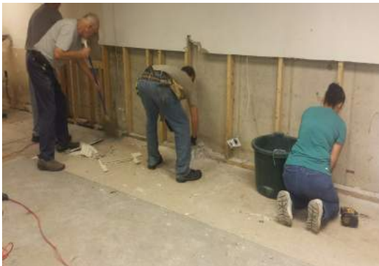
Contaminated drywall was gutted out to 42 inches above floor level.
